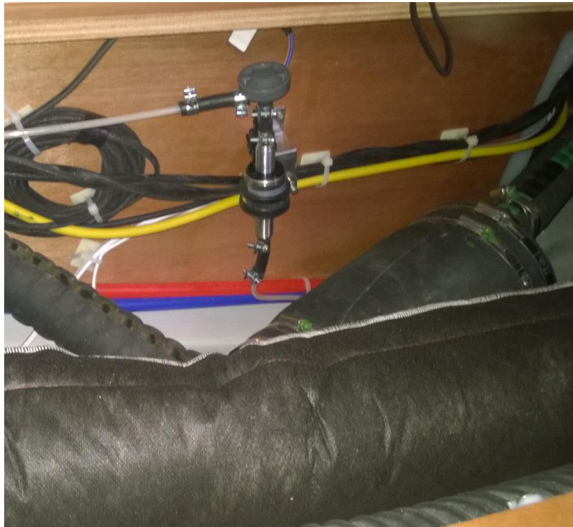
Figure 5 Pump and loom, insulated pipe in foreground
